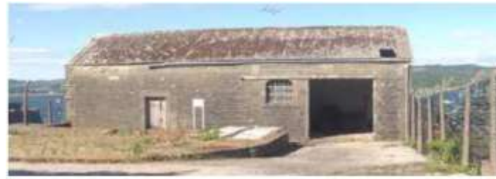
The 'Egg Shed', formerly used for storing dairy between sea, land and canal transportation
